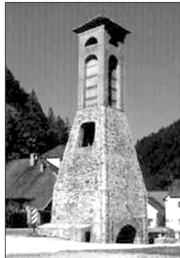
An old-fashioned iron smelting furnace from the north-western, ore-rich region of Slovenia, where metallurgy had been in use from the 14 th century to the beginning of the 20 th century.
